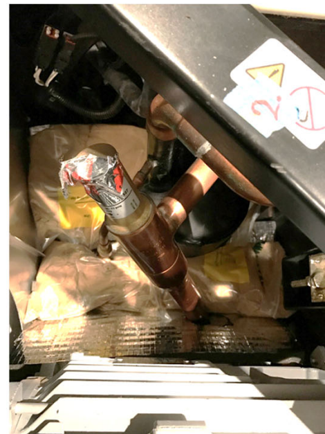
Sandbags on Power Tray
